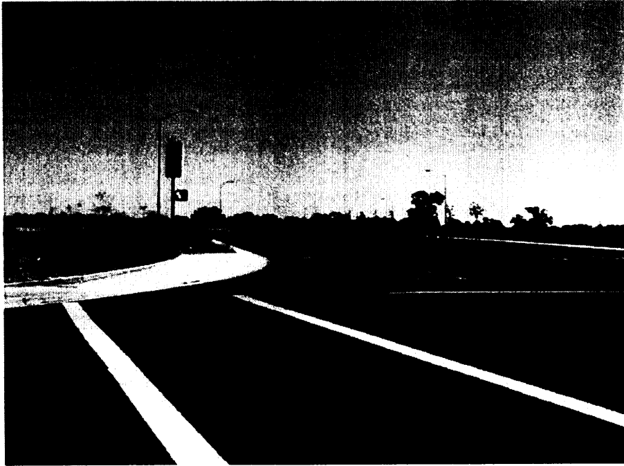
Looking southeasterly along Roseville Parkway
